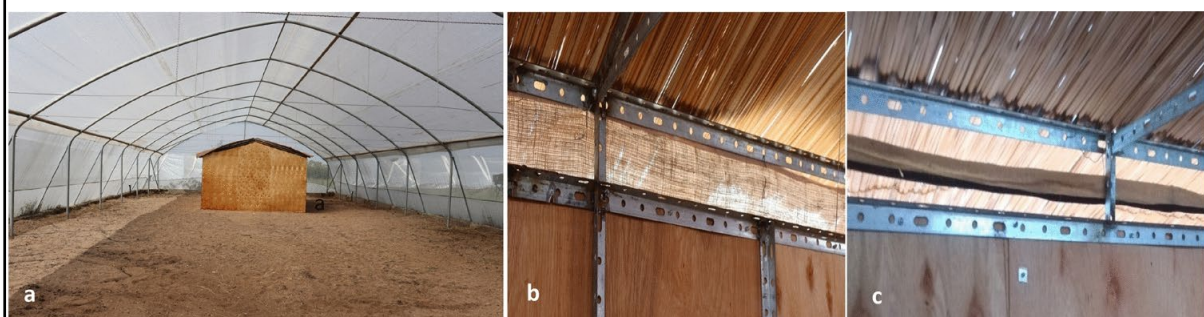
a Pictorial presentation of a semi-field system (27 m × 11 m), including an experimental hut made of plywood with a grass thatched roof (6.5 m × 3.5 m). b Application of an eave screen secured on the eave gap of the experimental hut using aluminium wires to ensure complete coverage of the eave gap ( c ) and eave strip secured on the eave gaps of the experimental hut using aluminium wires to ensure equal distance (2.5 cm) above and below the eave fabric
